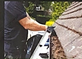
Gutter clearance & repairs
